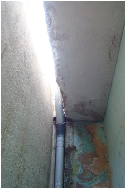
Fig. 2 S1 – Problem with drainage from upper floor and hygiene
