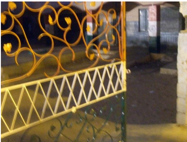
Figure 19. School gate left unlocked
