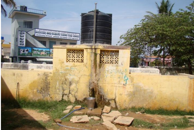
Figure 12. A typical rural school toilet facility
