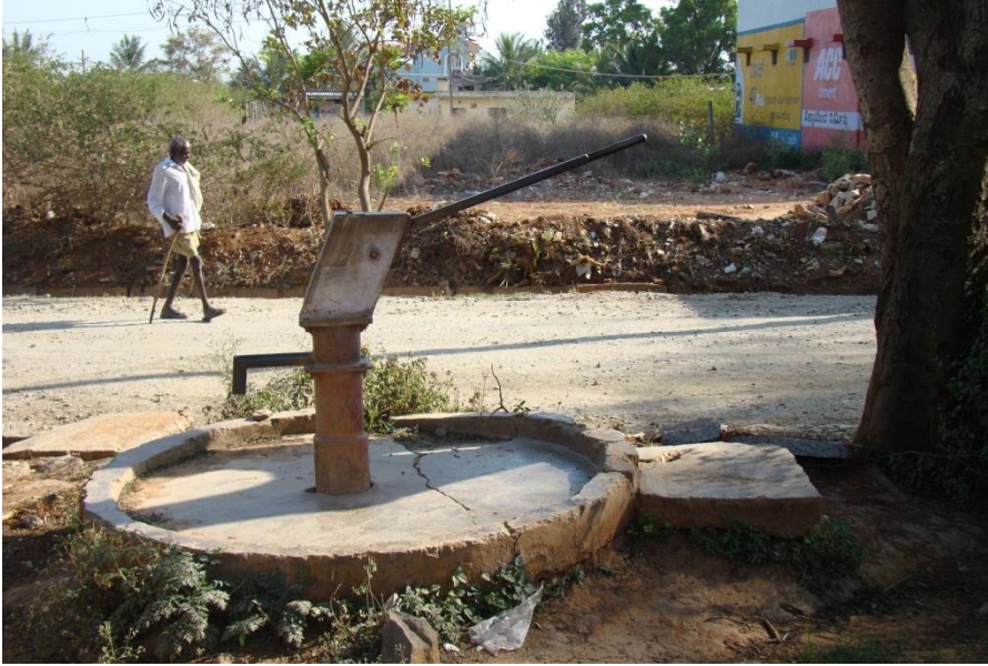
Figure 16. Rural water well pump
