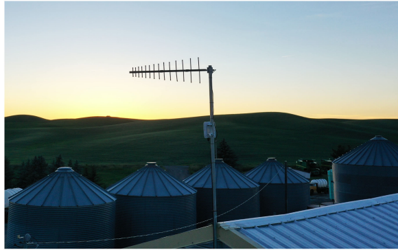
FIGURE 2. TV white space antenna and broadband radio in a farm in Eastern Washington.
